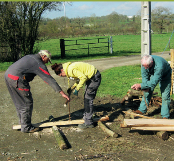
In Bressuire, project on the valuation of wooded heritage with construction of chestnut barriers (intergenerational).
